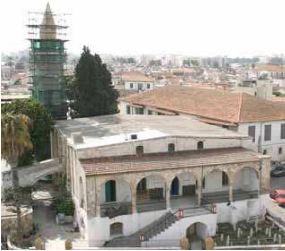
The Kebir Mosque in Lamaka under renovation.
