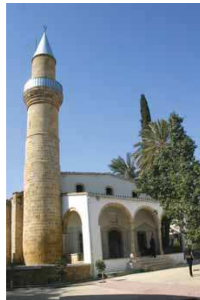
The completely renovated Mosque of Tahtakale in Lefkosia.
