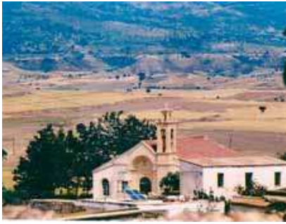
The Maronite church of Archangel Michael Asomatos was built in the centre of a village, bearing the same name.
