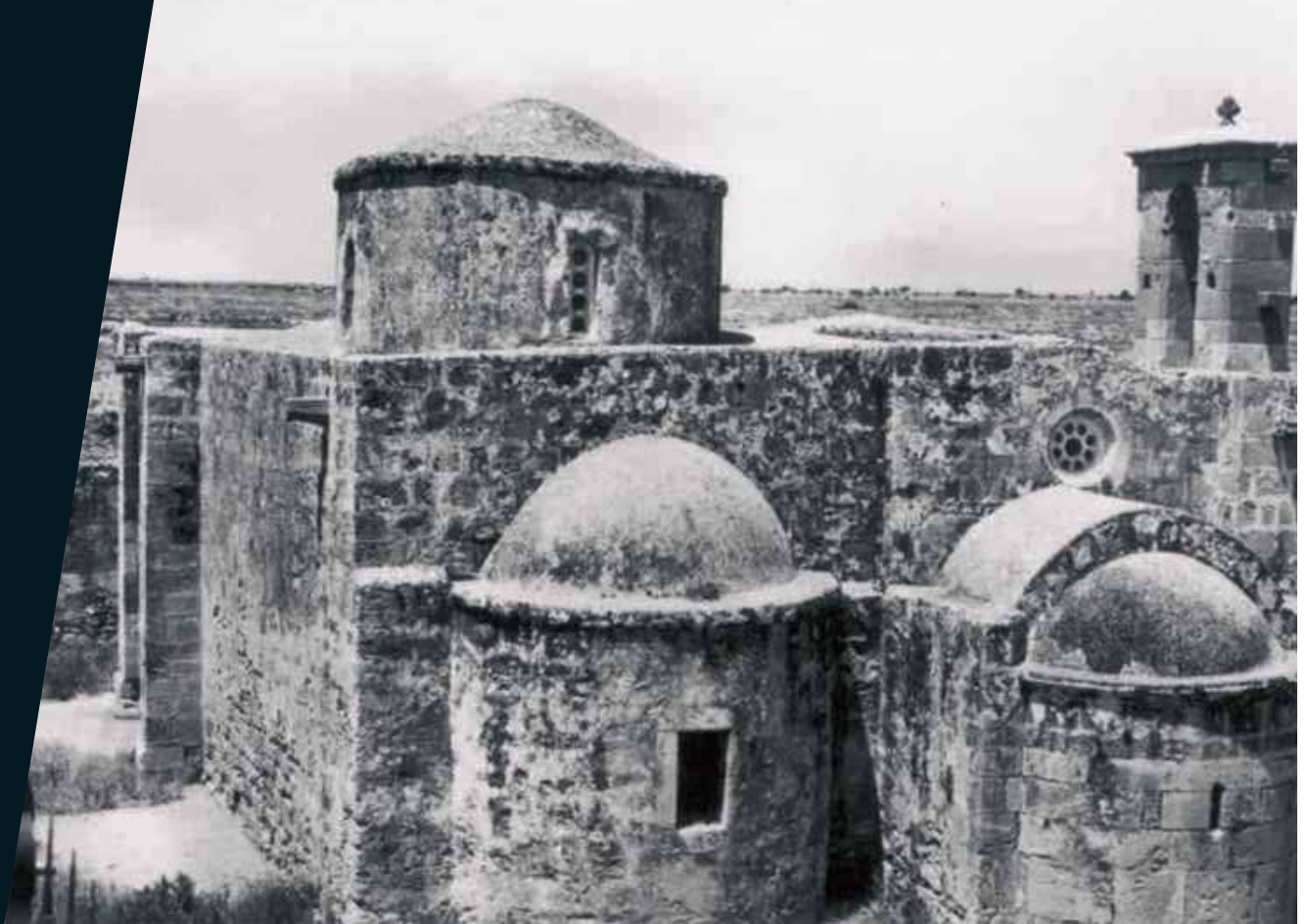
The medieval church of the monastery, as it was preserved until 1974.
