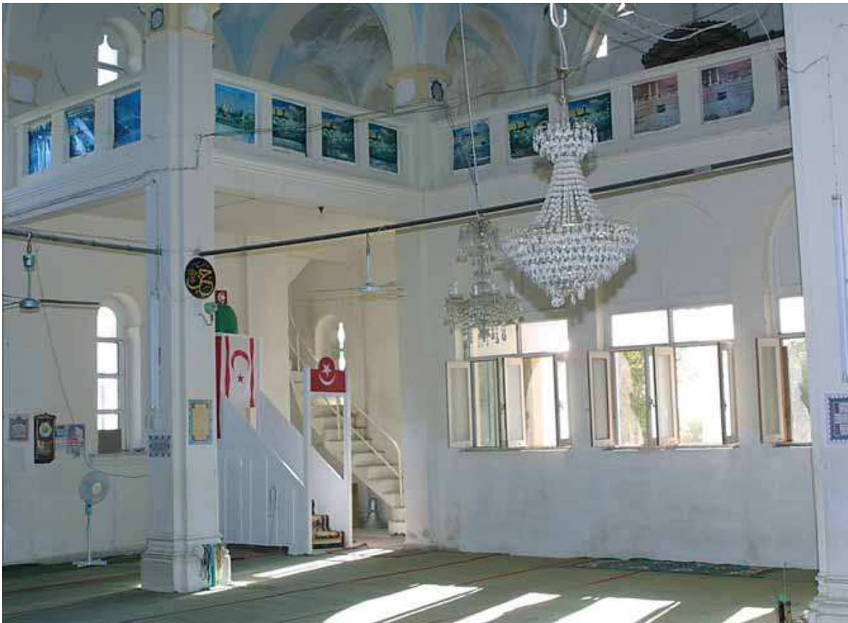
Detail of the west side of the church of St. Luke in Eptakomi, which was transformed into the mosque of the village.
