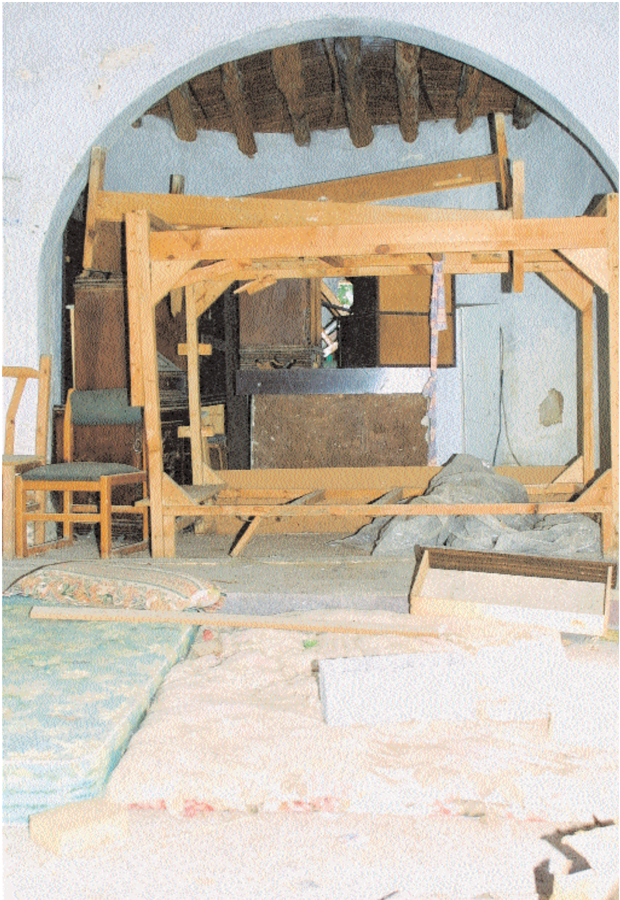
Interior view of former St. George church in Spathariko. Mattresses and furniture can be seen in what is now a private home.
