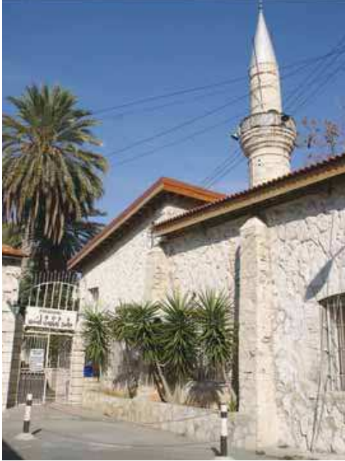
The Kebir Mosque in Lemesos undergoing total renovation.
