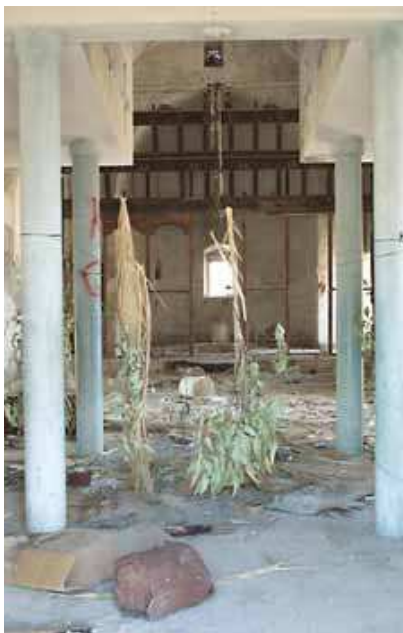
Abandoned and destroyed Church of St. George in Afanteia.
